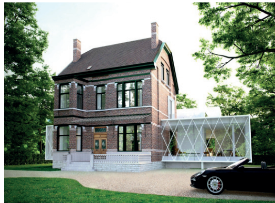
Kanoor immoflandria, Melle: Caan architecten
